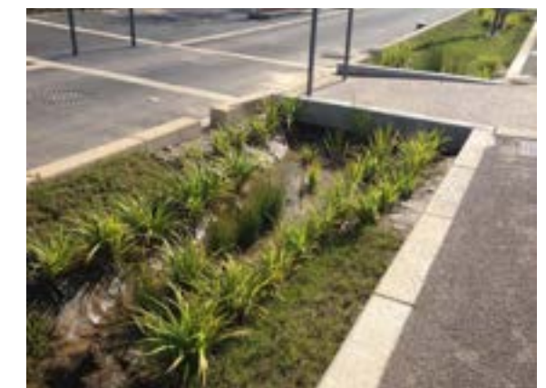
PHOTO 30: GREEN DRAINAGE BED, DOUAI, FRANCE
