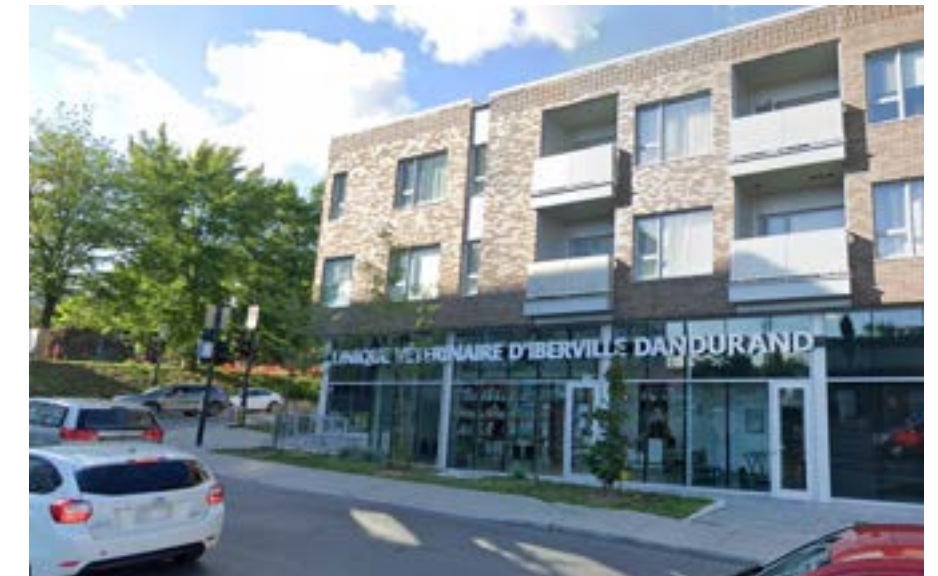
PHOTO 24: GROUND FLOOR COMMERCIAL SPACES WITH HIGH CEILINGS
