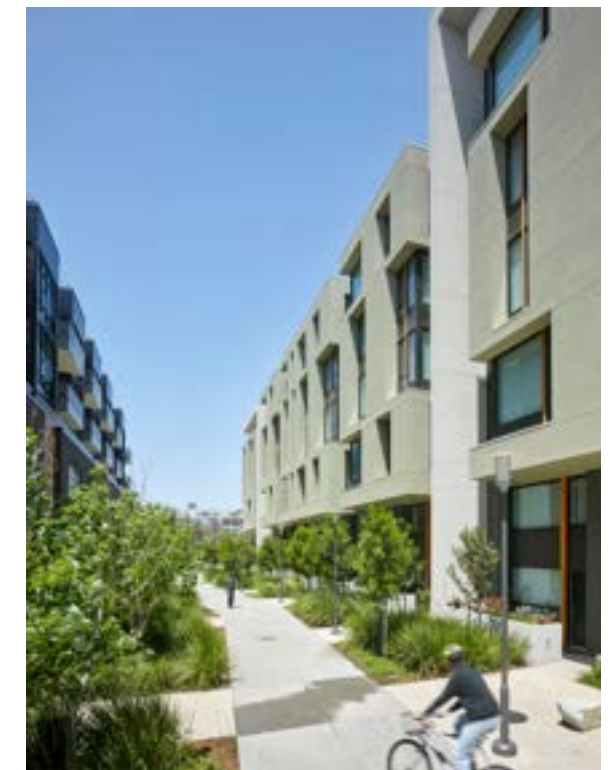
PHOTO 26: 1180, 4TH STREET, SAN FRANCISCO - QUALITY CONTEMPORARY ARCHITECTURE LOCATED ON A PROMENADE
