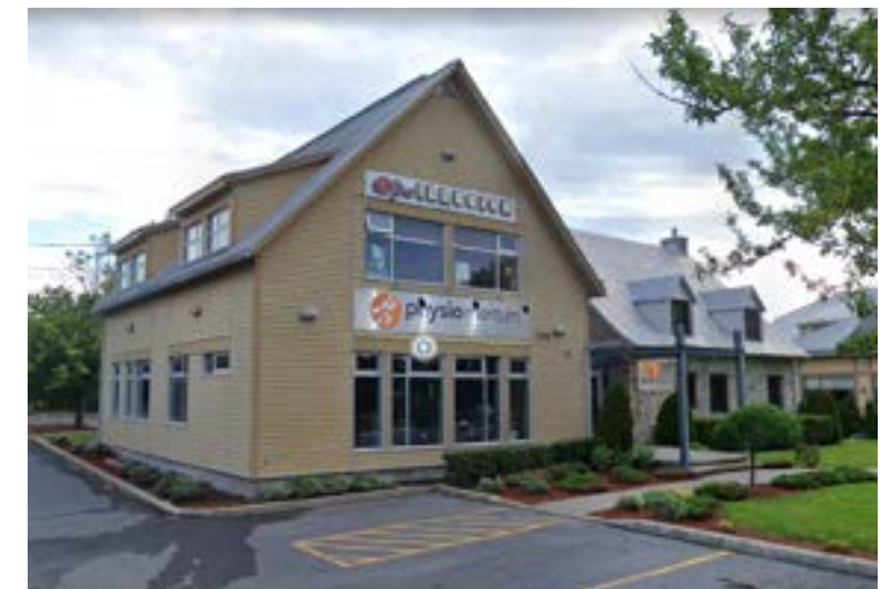
PHOTO 5: JOSEPH-RABEAU RESIDENCE IN ITS CURRENT FORM
