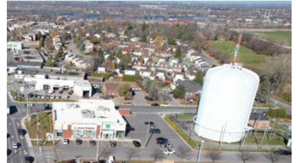
PHOTO 22: WATER RESERVOIR AT THE ST. CHARLES PUMPING STATION
