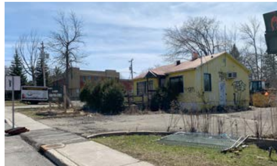
PHOTO 18: BUILDING THAT NEEDS TO BE RENOVATED
