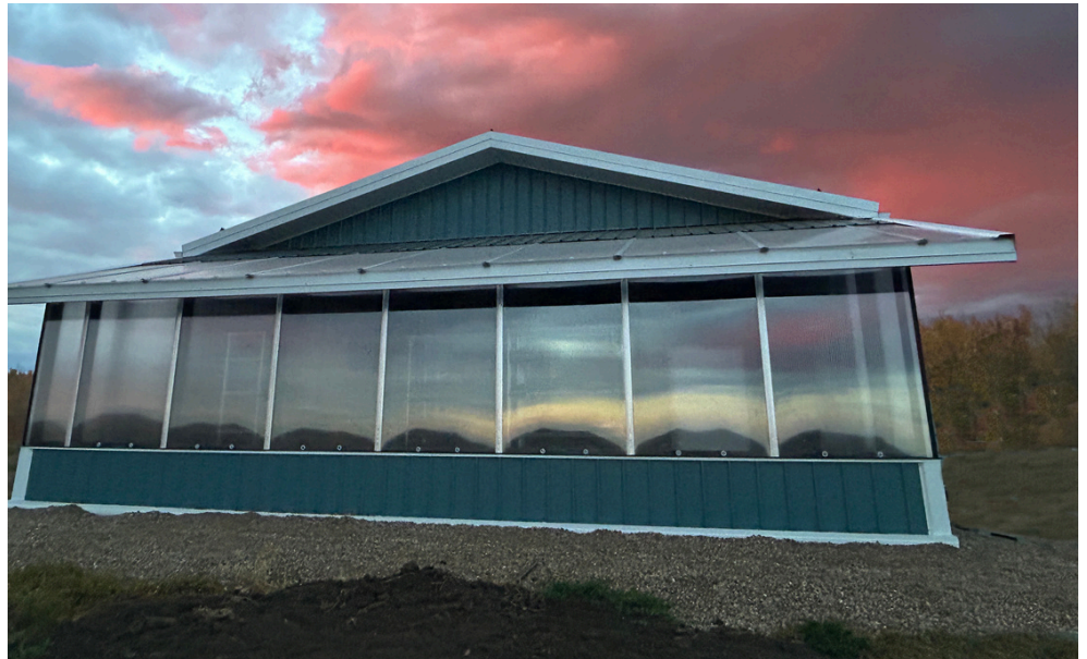
Kross Farms Passive Solar Greenhouse in Manville, AB.
