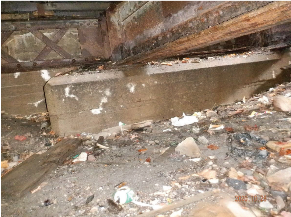
South abutment wall
