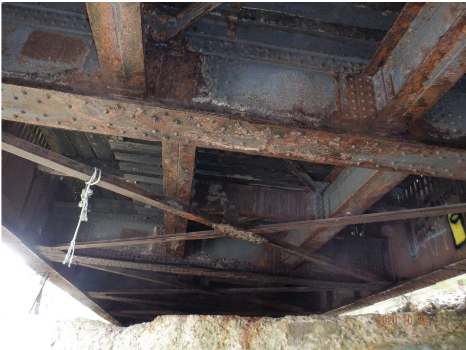
South span soffit
