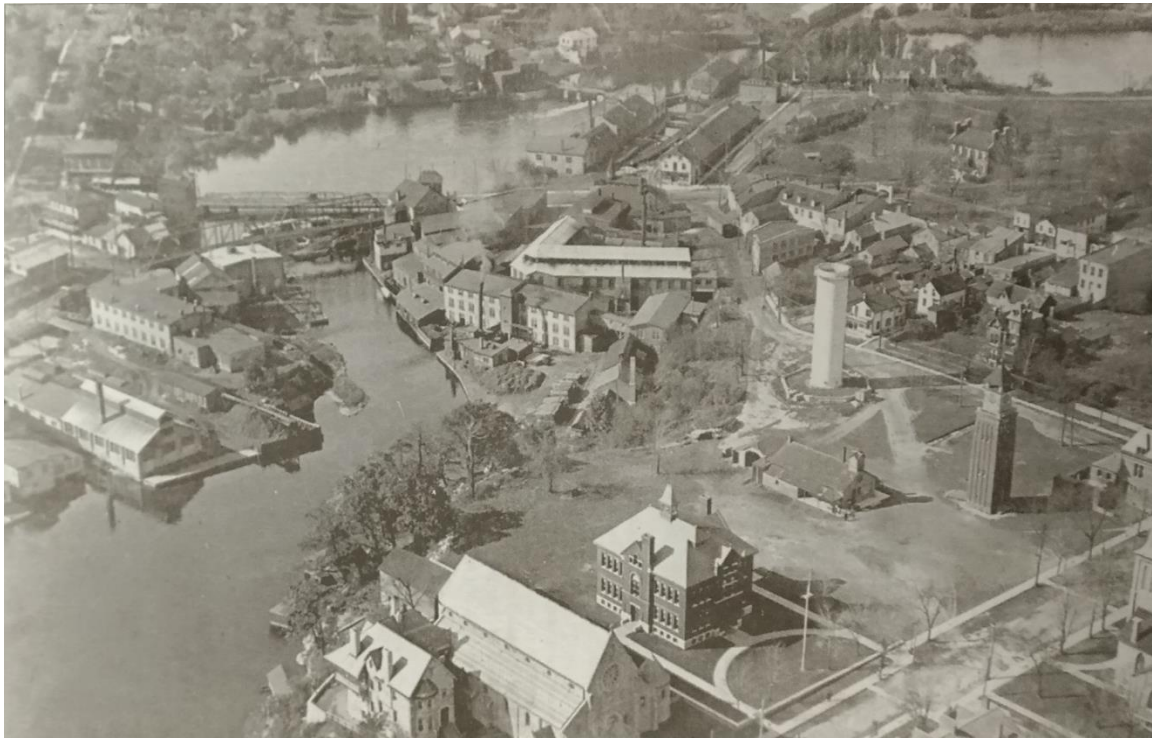
Figure 26: Oblique aerial view of Market Square, 1919 showing St. John's from the southeast, the former High School is to the immediate right/north, then the low fire hall, then the clock/hose drying tower to its right/northeast and the cylindrical former water tower to the firehall's northwest (Gananoque Historical Society Newsletter, no. 38, Sept. 2002, p. 951).
