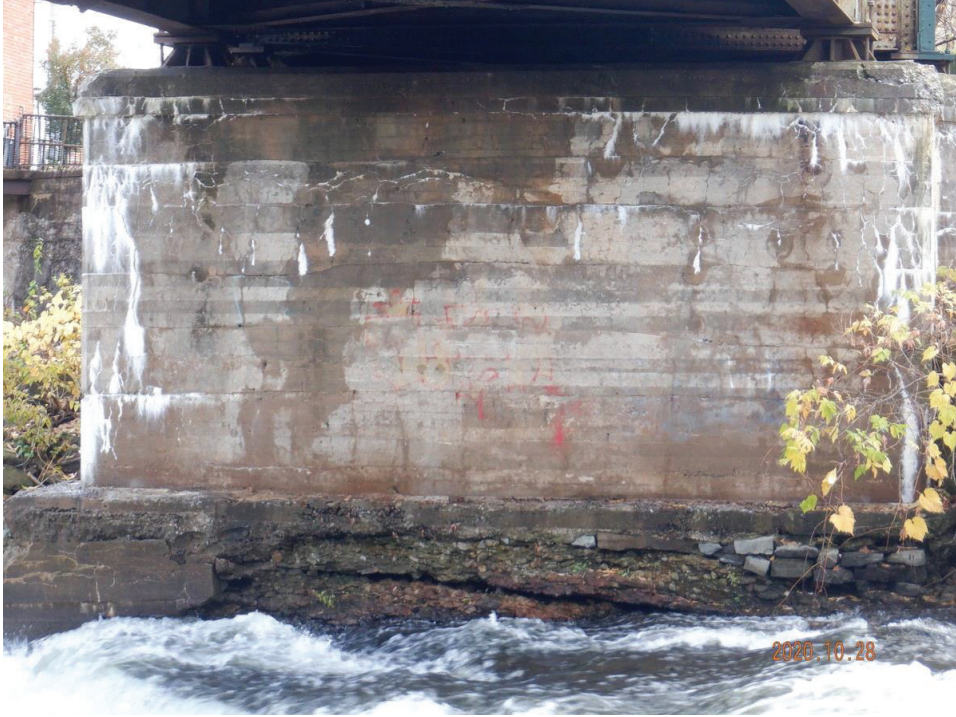
North face of pier
