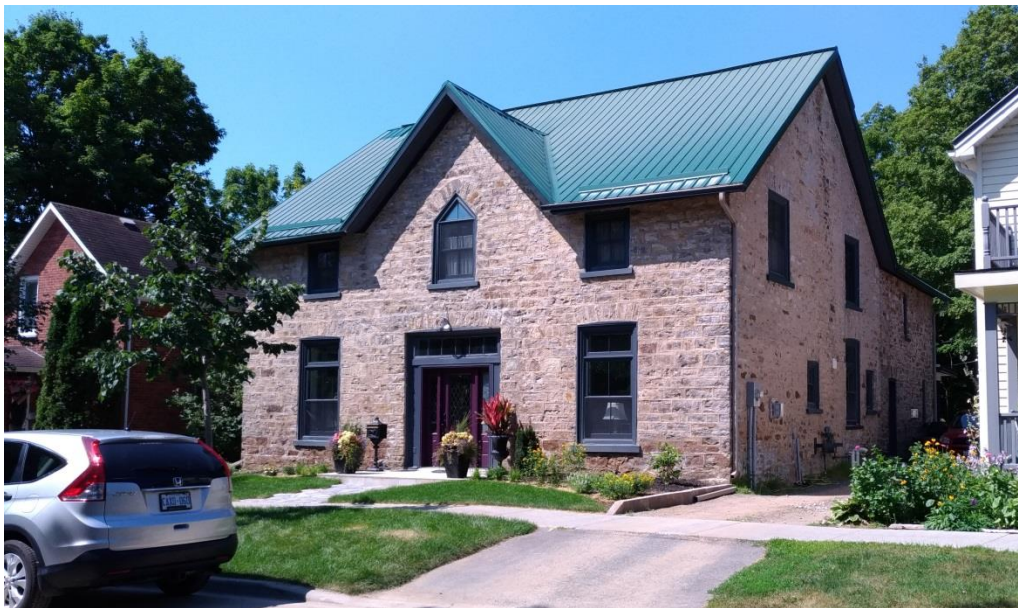
Figure 7: 40 Princess St., the first Christ Church Rectory, viewed from the northeast, built after the first phase of Christ Church 1857-58, enlarged at the rear late 1910s (photo E. Tumak, July 2009).
