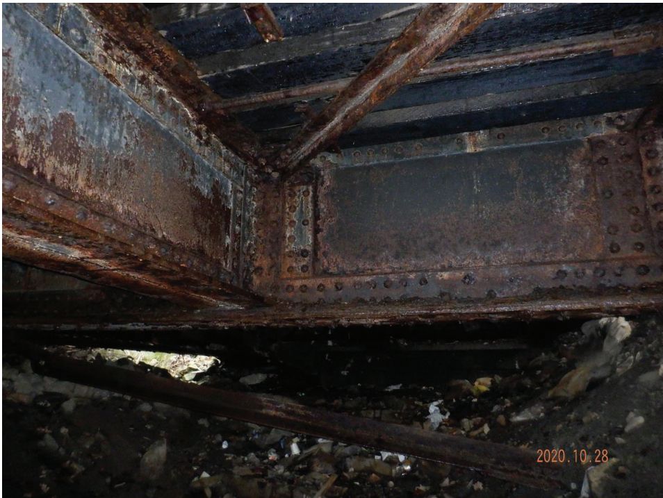
South floor system condition
