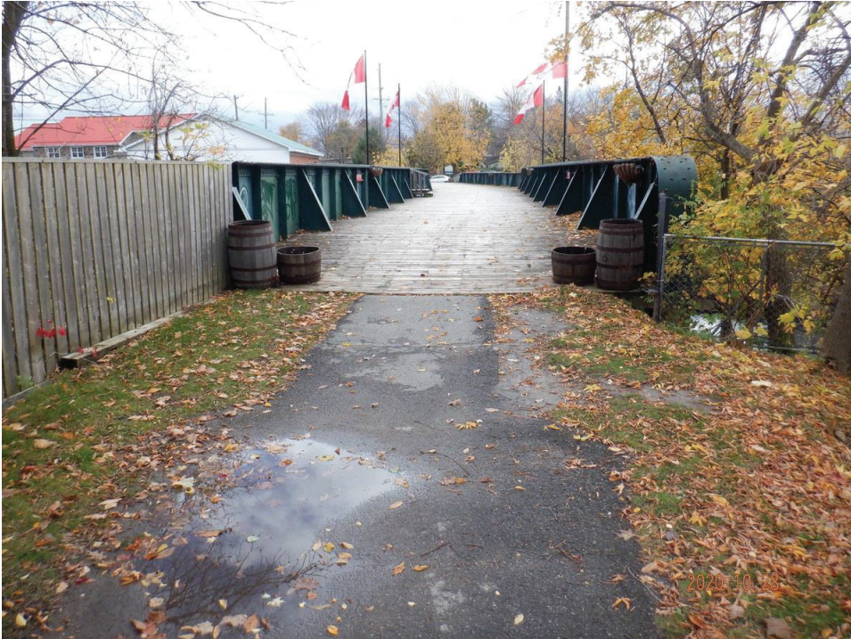
Looking south over bridge
