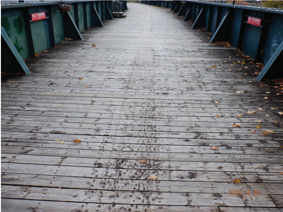
Wearing surface over bridge
