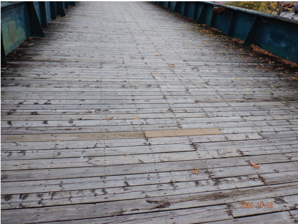
Deck wearing surface
