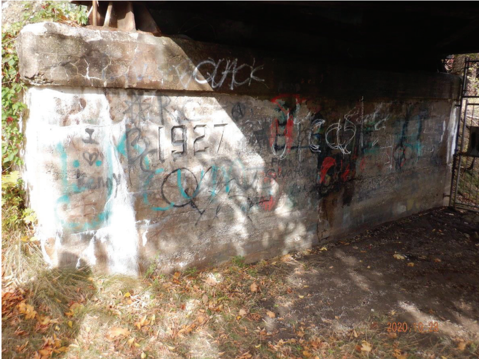
North abutment wall
