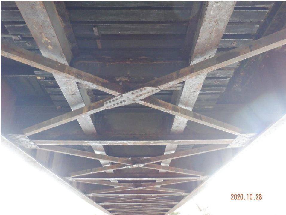
North span soffit
