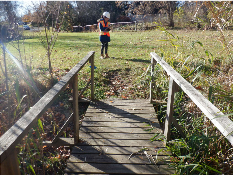
Figure 4 : Bridge Looking West
