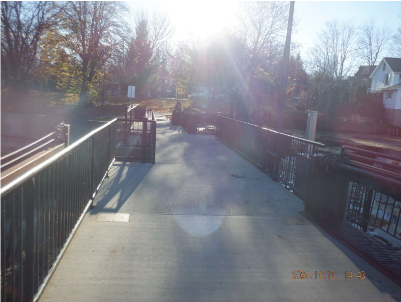
Figure 4 : Bridge Looking South
