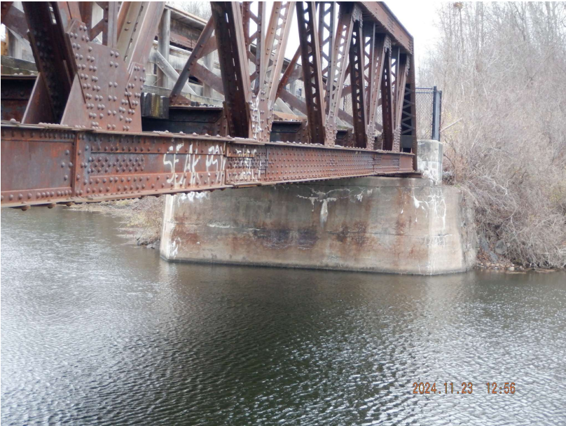
Figure 12 : North Abutment (Typ.)
