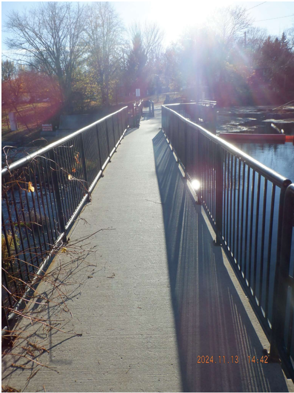
Figure 7 : Bridge Deck (Typ.)
