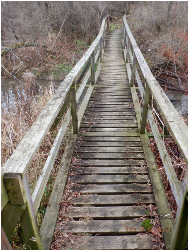
Figure 8 : Bridge Deck (Typ.)
