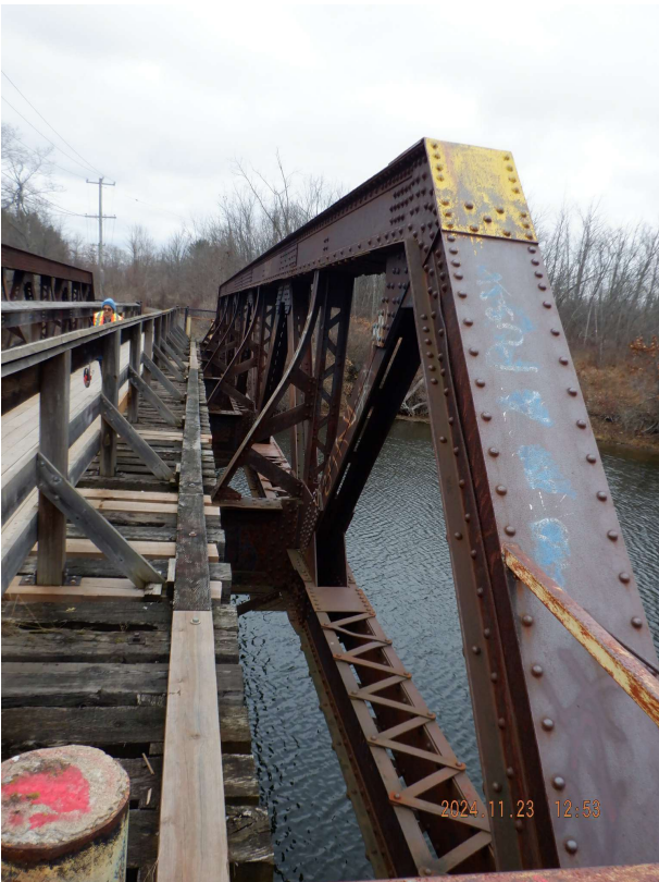
Figure 10 : Original Bridge Truss (Typ.)
