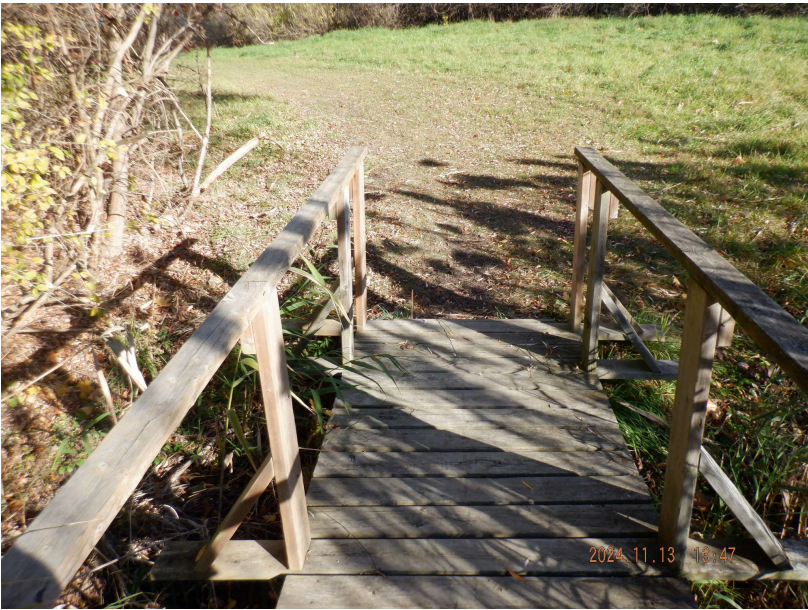
Figure 3 : Bridge Looking East
