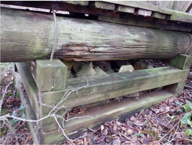
Figure 19 : East Abutment Crib (Typ.)
