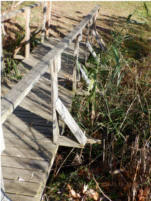
Figure 10 : Railing Post Connection Detail (Typ.)
