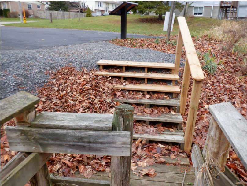
Figure 4 : West Approach & Staircase
