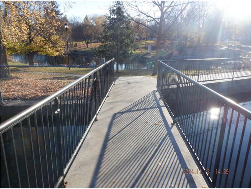
Figure 4 : Bridge Looking South
