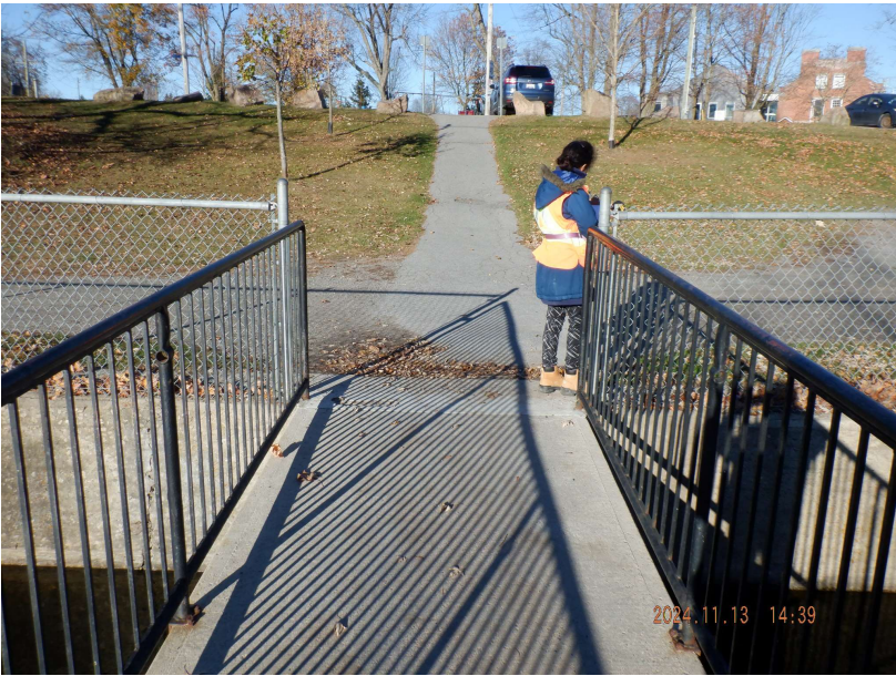
Figure 3 : Bridge Looking North
