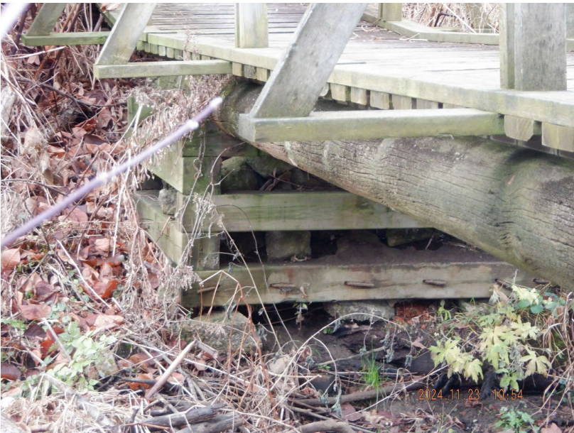
Figure 20 : West Abutment Crib (Typ.)
