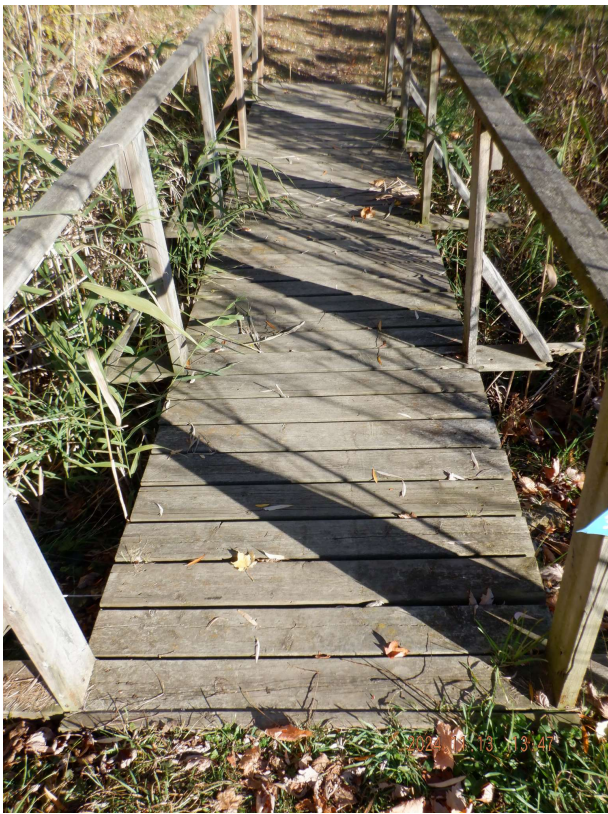
Figure 7 : Deck Condition (Typ.)
