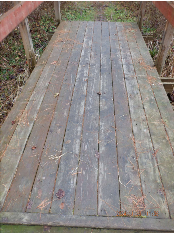
Figure 6 : Bridge Deck (Typ.)
