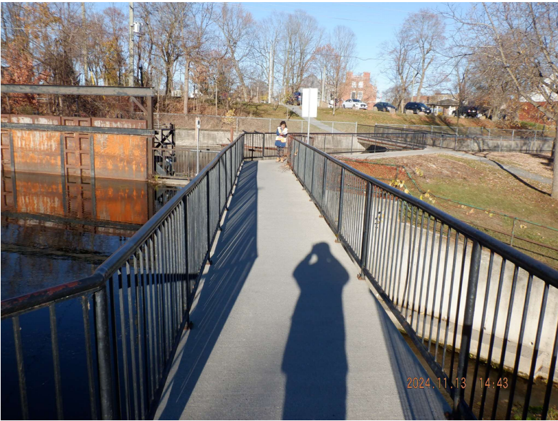
Figure 3 : Bridge Looking North
