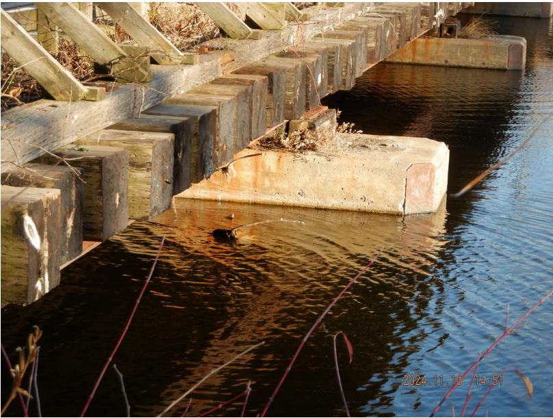
Figure 11 : Pier Foundation (Typ.)
