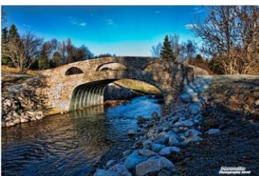
Figure 4 Stone Bridge in Bowring Park after Restoration
