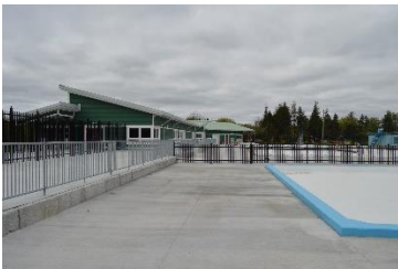
Figure 7 Pool House in Bowring Park
