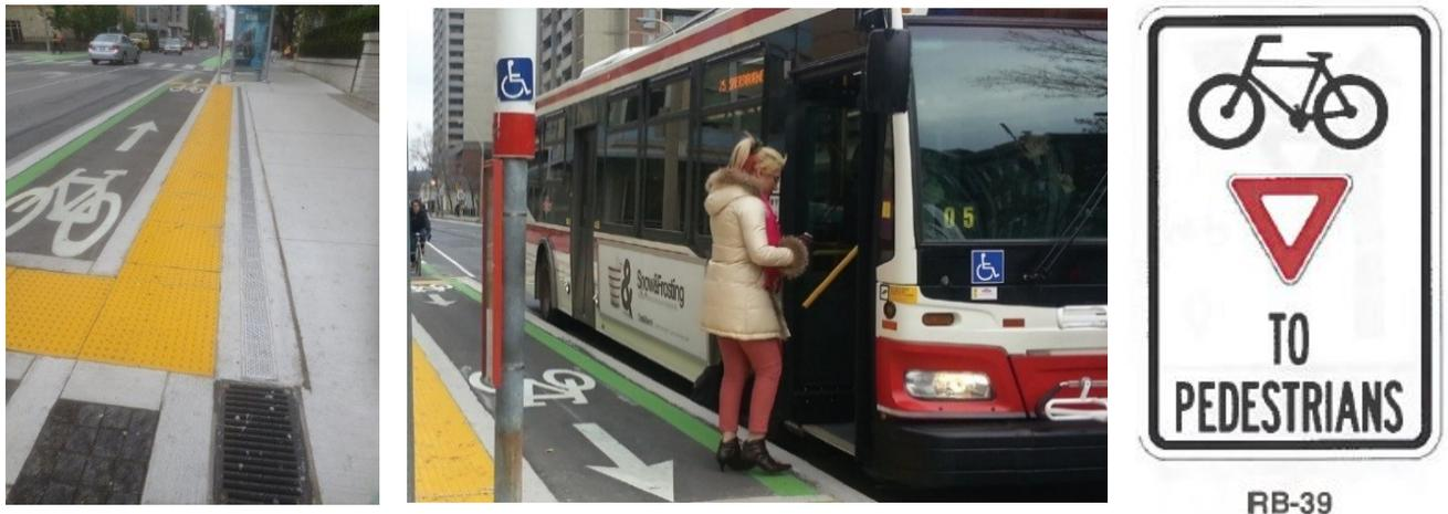
Figures 2.1 – 2.3: Examples of a shared bus stop-raised bike lane treatment from Sherbourne Street (Toronto), Roncesvalles (Toronto), and an example of signage produced by Transportation Association of Canada.
