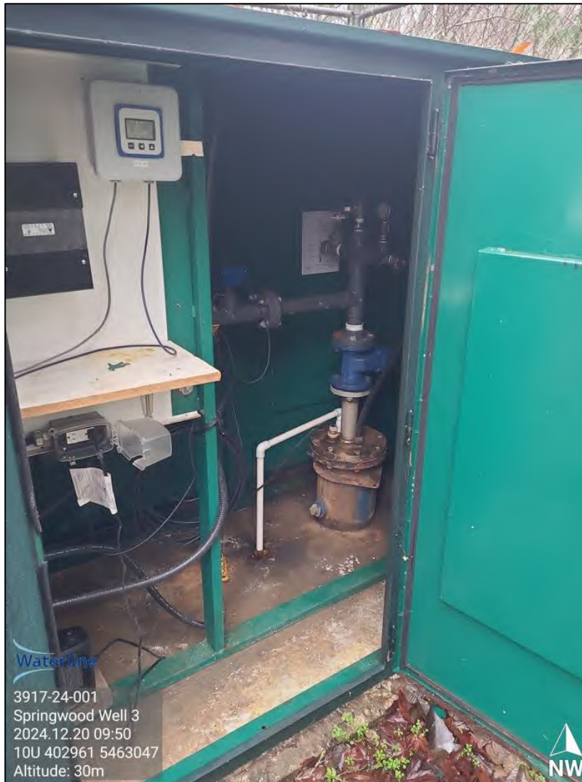
Photograph A11 (LEFT): SW 3 – Looking inside the well house, no issues noted. The well is flowing artesian during periods of non-pumping. Photograph A12 (RIGHT): SW 3 – Close-up view of the wellhead. The flowing water is being directed to a floor drain.
