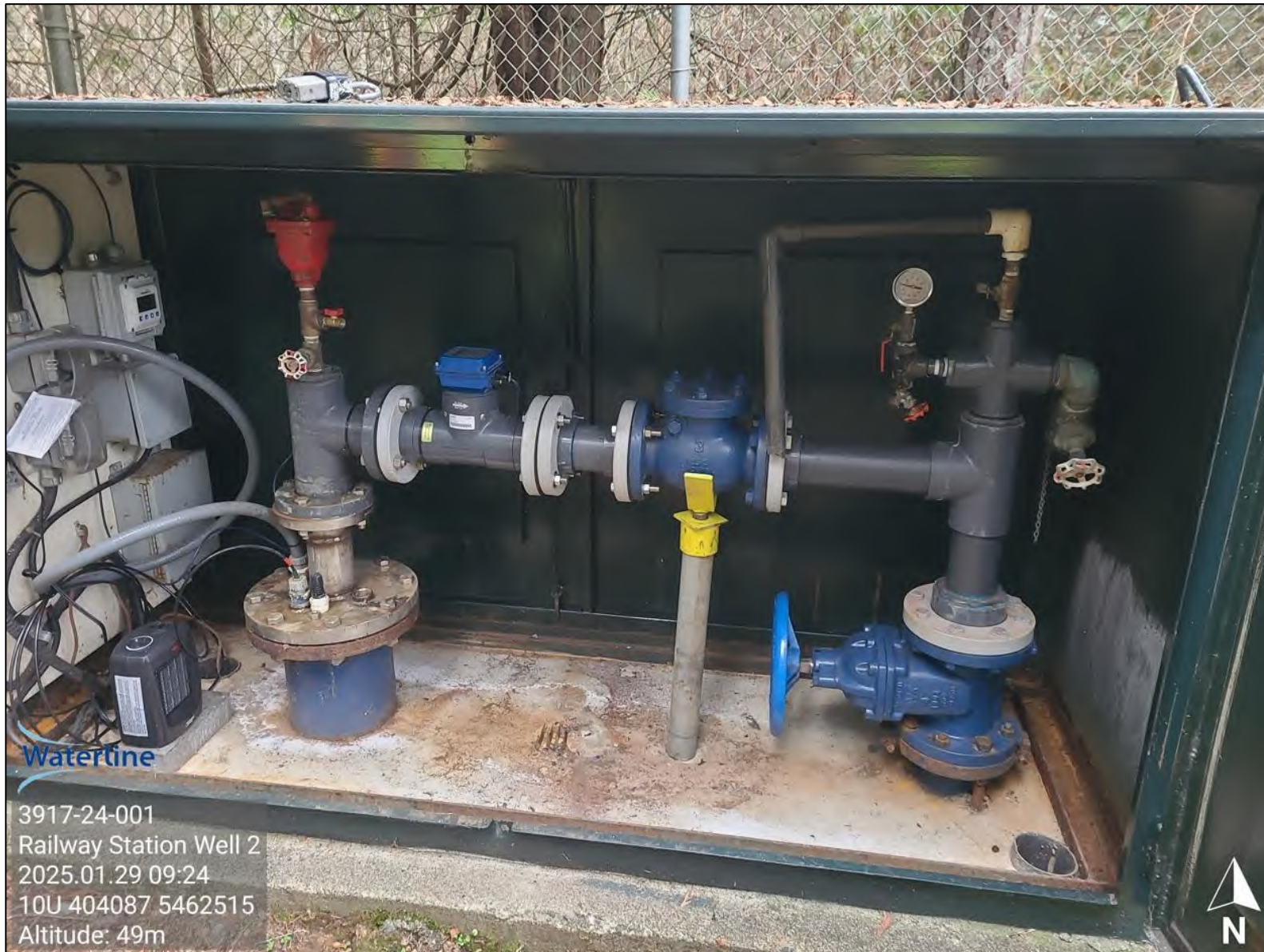
Photograph A2: RSW 2 – Looking inside the well house. No issues noted.
