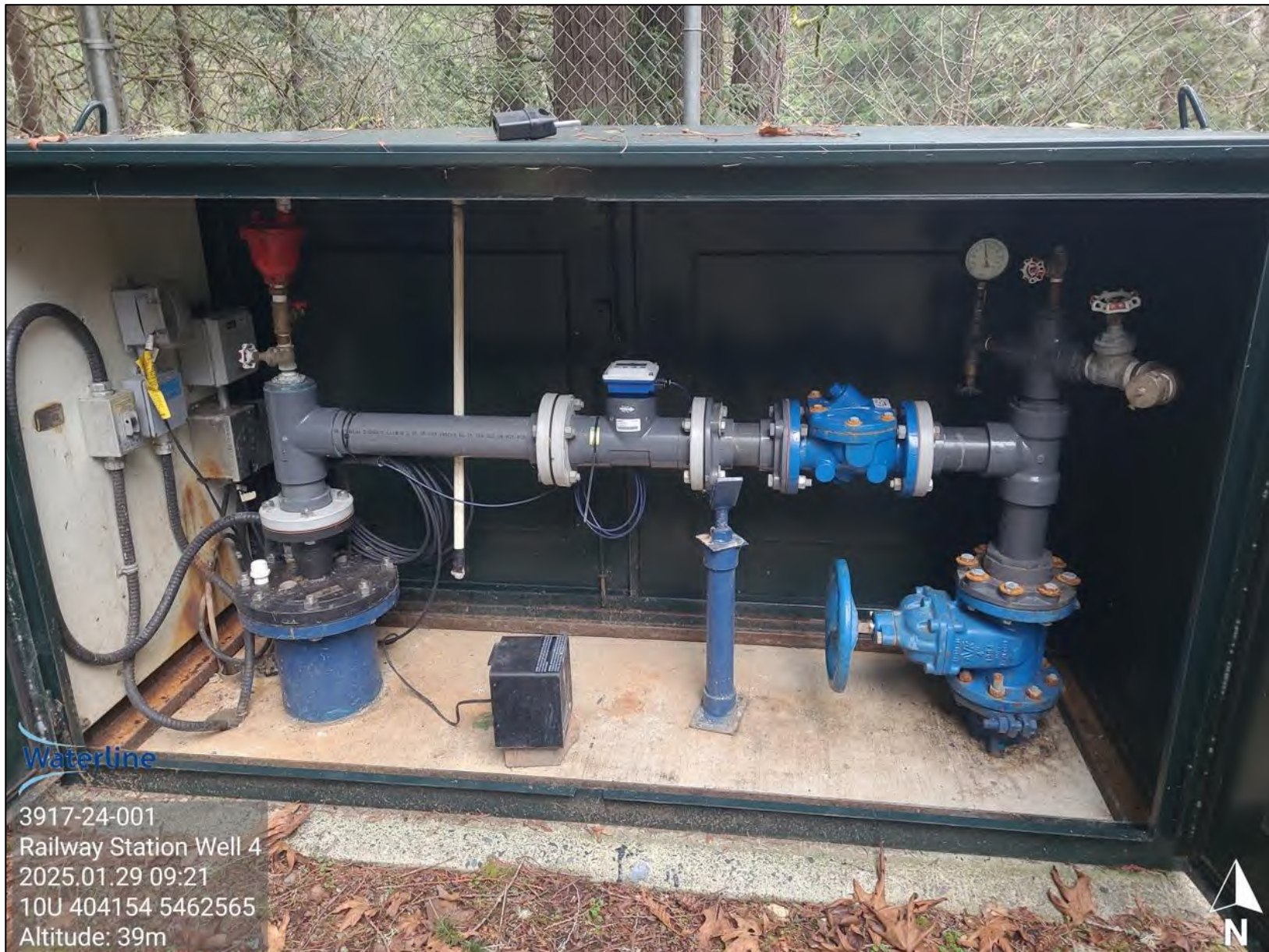
Photograph A4: RSW 4 – Looking inside the well house. No issues noted.
