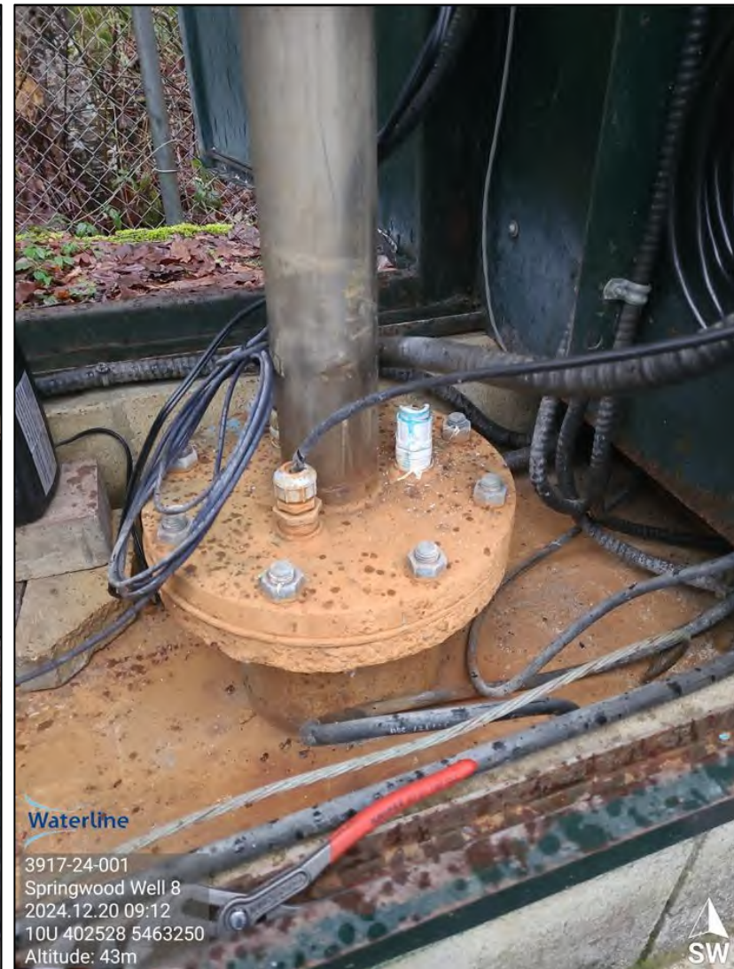
Photograph A17 (LEFT): SW 8 – Looking inside the well house. No issues noted. Photograph A18 (RIGHT): SW 8 – Close-up view of the wellhead. The well can exhibit intermittent flowing artesian conditions during periods of non-pumping and therefore, a 1" PVC pipe is installed to direct flow towards a floor drain.
