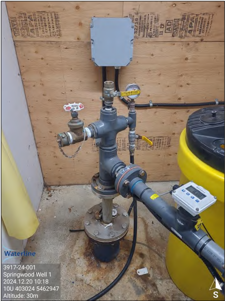
Photograph A8 (LEFT): RSW 8 – Looking down at the wellhead. No issues noted. Photograph A9 (MIDDLE): SW 1 – Looking down and south at the wellhead. Photograph A10 (RIGHT): SW 1 – Looking down and north at the wellhead. The electrical cable for the pump, that is passing through the well house floor (concrete) inside a PVC conduit, is not secured (unsealed).
