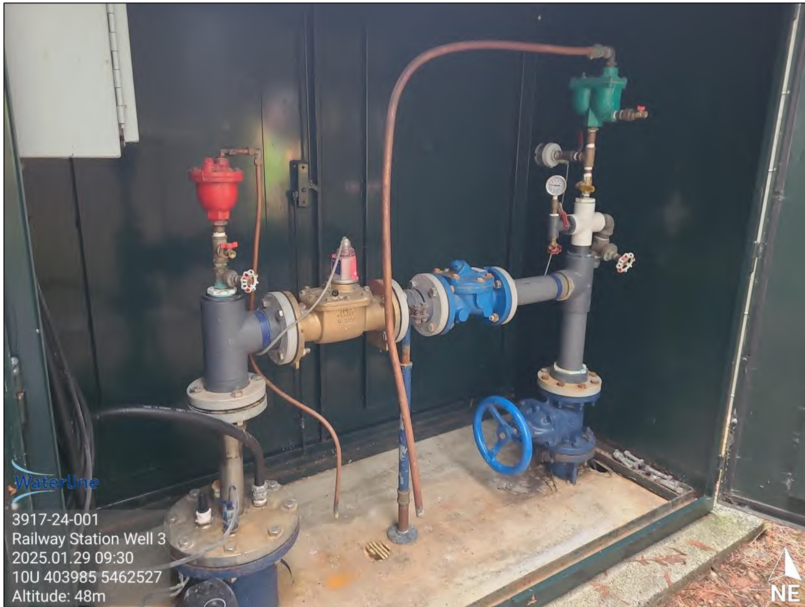
Photograph A3: RSW 3 – Looking inside the well house. No issues noted.
