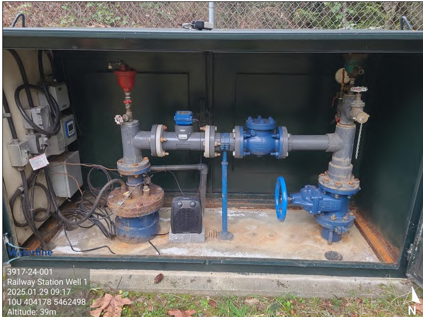
Photograph A1: RSW 1 – Looking inside the well house. No issues noted.
