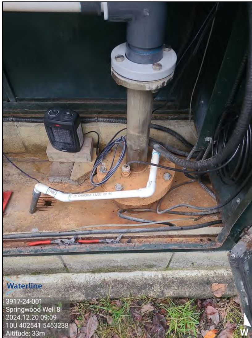
Photograph A17 (LEFT): SW 8 – Looking inside the well house. No issues noted. Photograph A18 (RIGHT): SW 8 – Close-up view of the wellhead. The well can exhibit intermittent flowing artesian conditions during periods of non-pumping and therefore, a 1" PVC pipe is installed to direct flow towards a floor drain.
