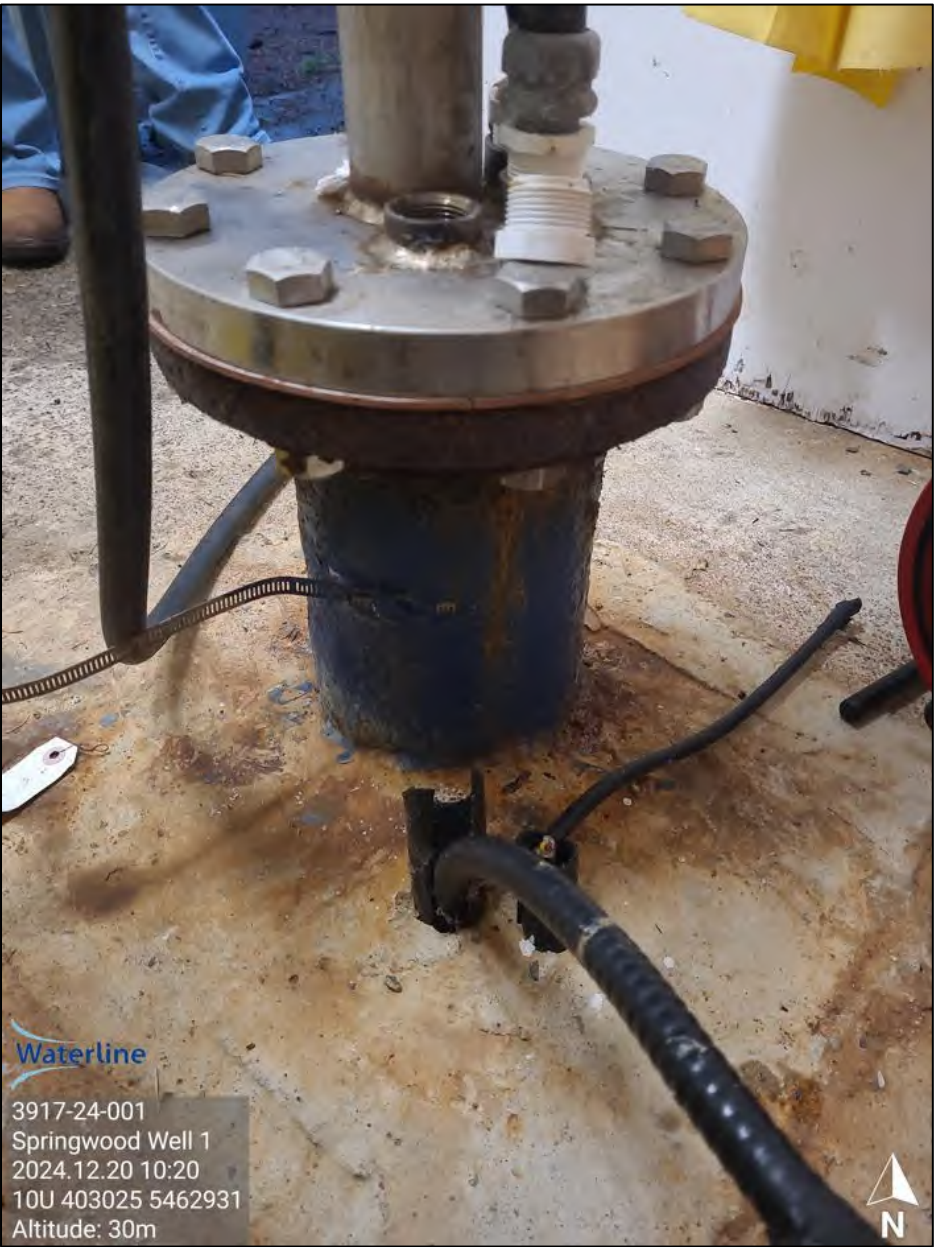
Photograph A8 (LEFT): RSW 8 – Looking down at the wellhead. No issues noted. Photograph A9 (MIDDLE): SW 1 – Looking down and south at the wellhead. Photograph A10 (RIGHT): SW 1 – Looking down and north at the wellhead. The electrical cable for the pump, that is passing through the well house floor (concrete) inside a PVC conduit, is not secured (unsealed).
