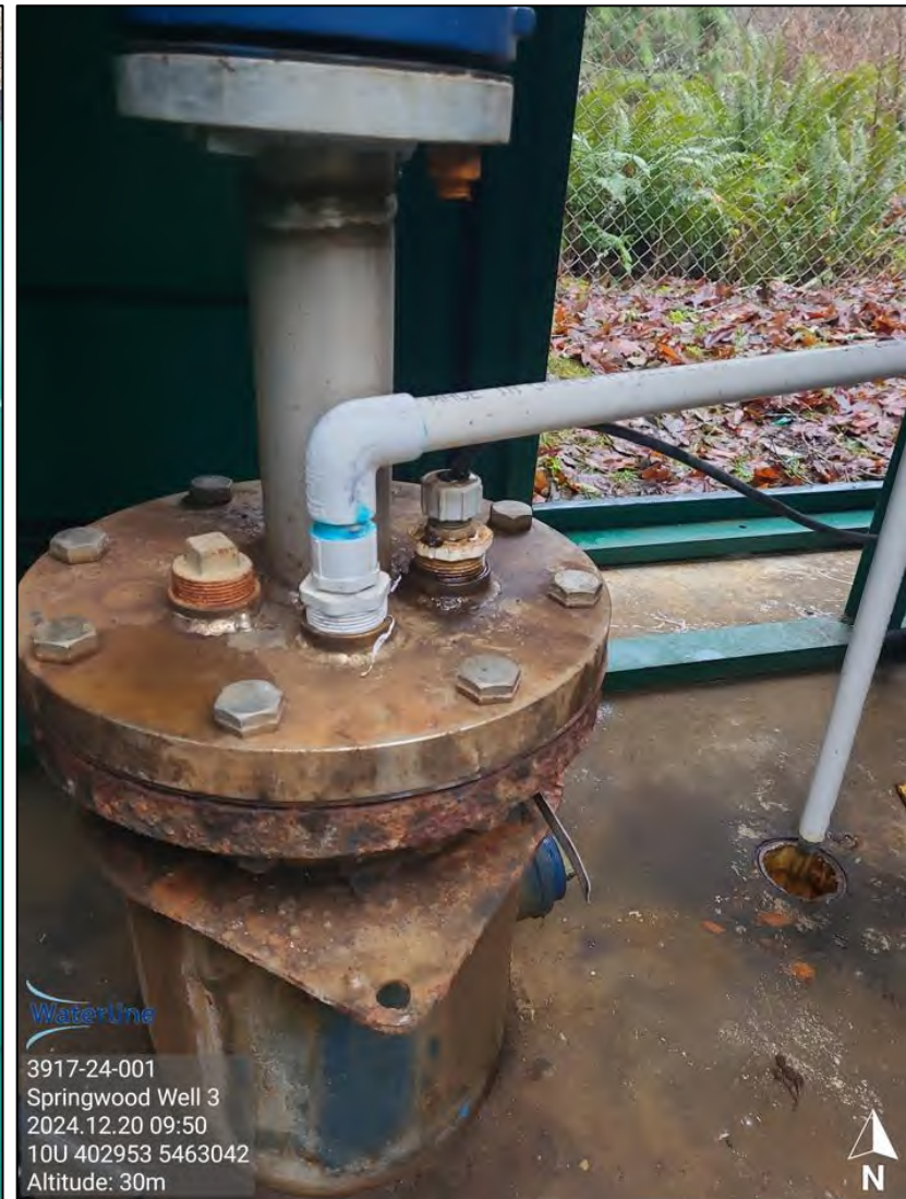
Photograph A11 (LEFT): SW 3 – Looking inside the well house, no issues noted. The well is flowing artesian during periods of non-pumping. Photograph A12 (RIGHT): SW 3 – Close-up view of the wellhead. The flowing water is being directed to a floor drain.
