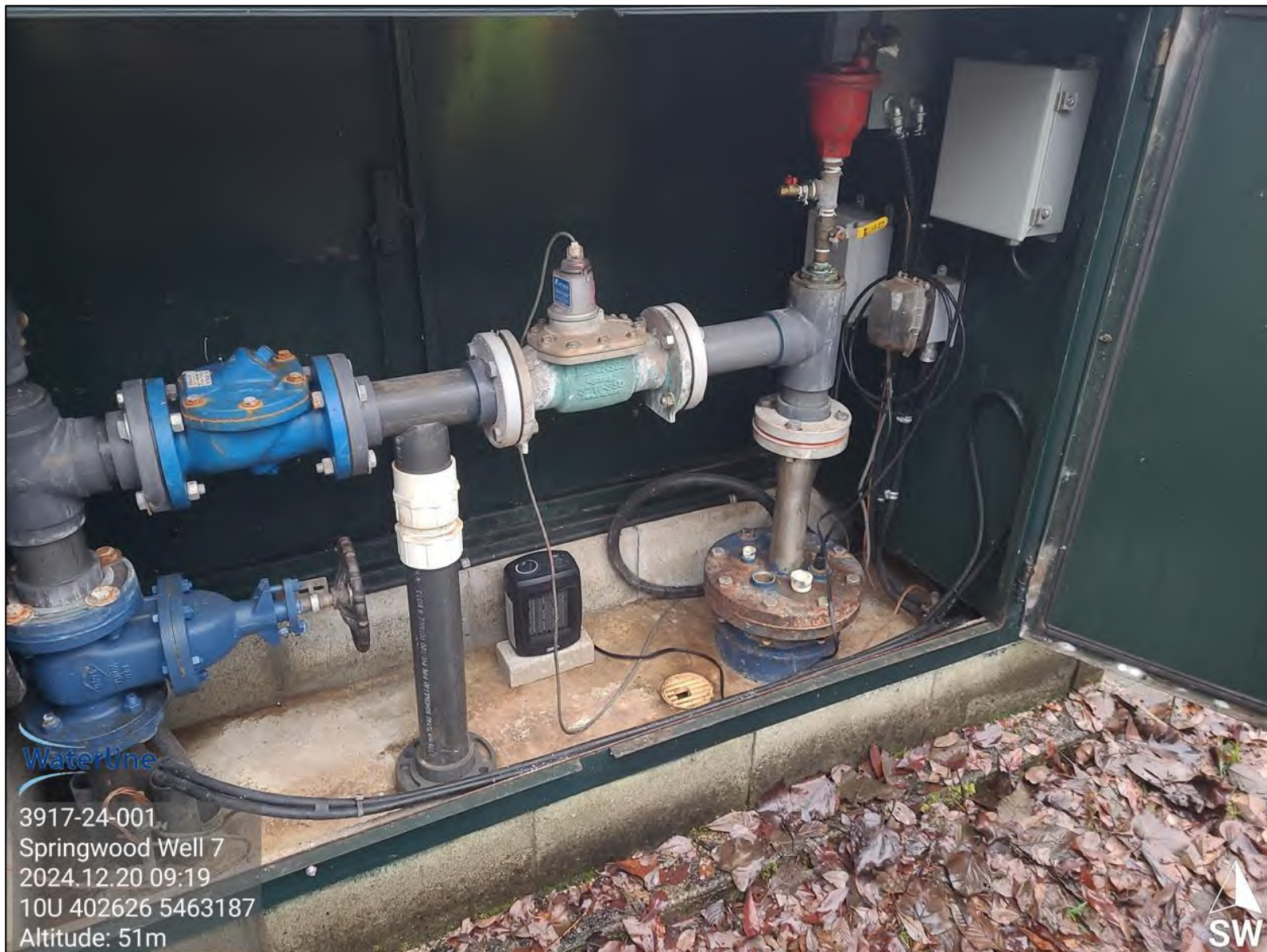
Photograph A16: SW 7 – Looking inside the well house. No issues noted. The well can exhibit intermittent flowing artesian conditions during periods of non-pumping.
