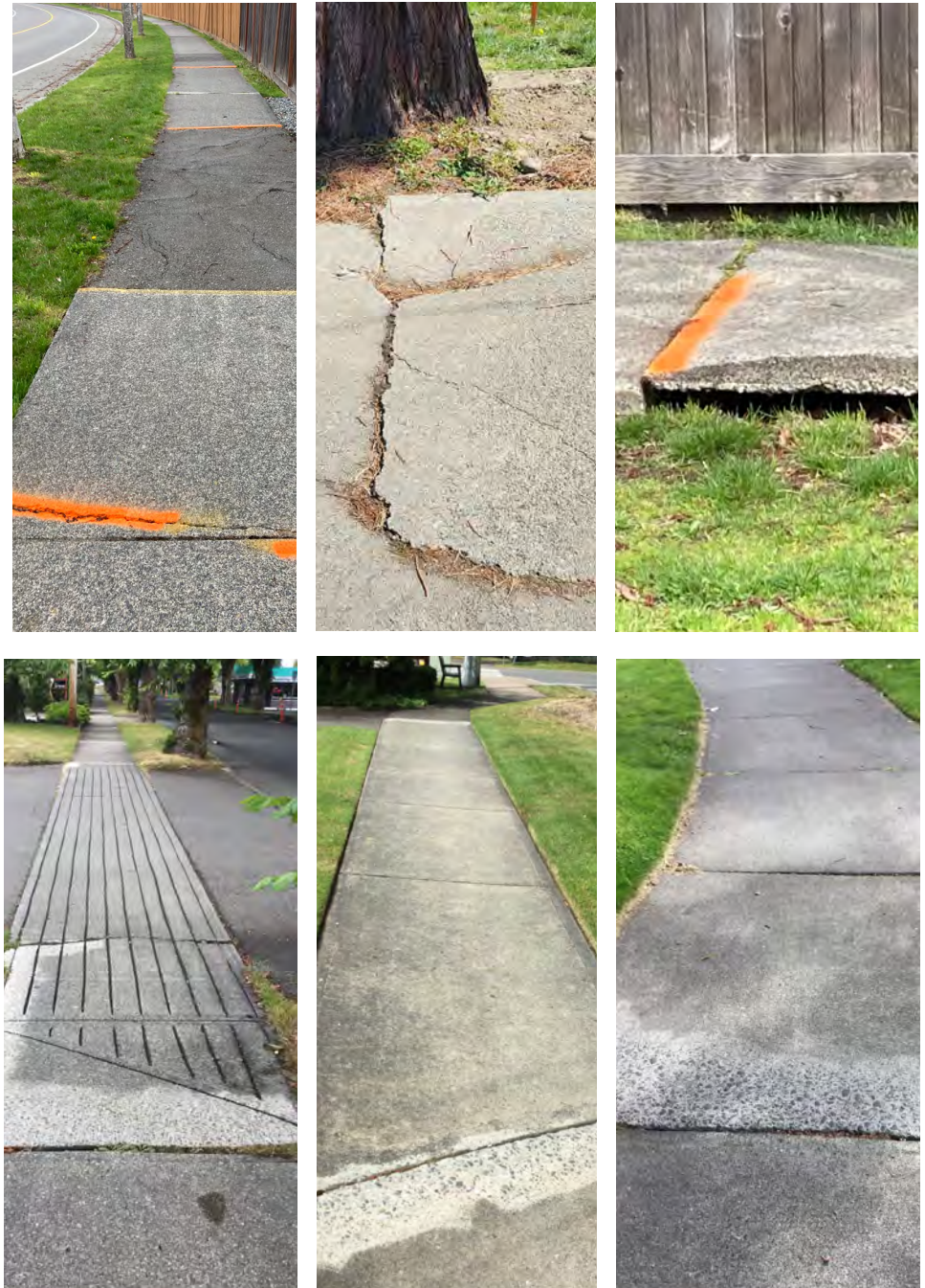
Figure 19. Examples of sidewalk conflicts (left) with trees (top) and responsive solutions (beveling, bottom).
